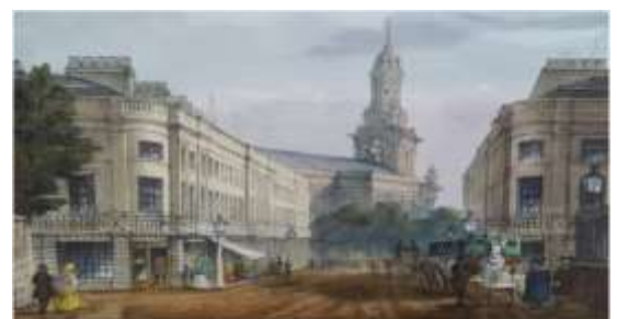
An early-Victorian view of Nelson Road, Greenwich, showing light-coloured stucco upper storeys and shop-front divisions and dark painted window joinery
